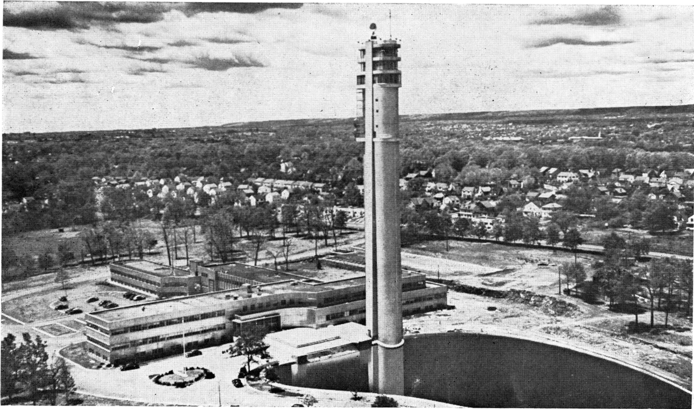
Federal Telecommunication Laboratories with 300-foot Microwave Research Tower
